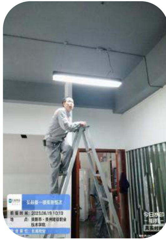
弘毅楼一楼照明整改
